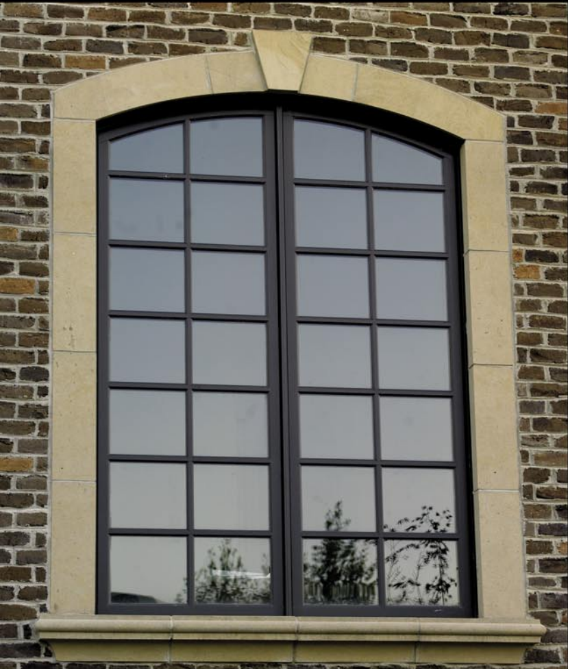
TWEED SANDSTONE WINDOW SURROUND
