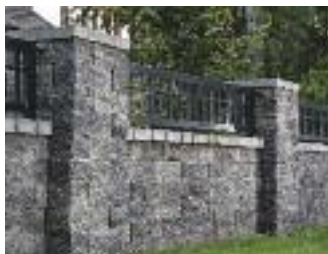
AB Courtyard Wall and Post Caps
