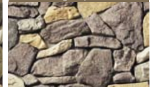
Tight-Fitted Mortar Joints
