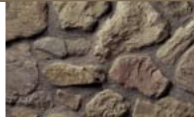
Wide Mortar Joints, Raked
